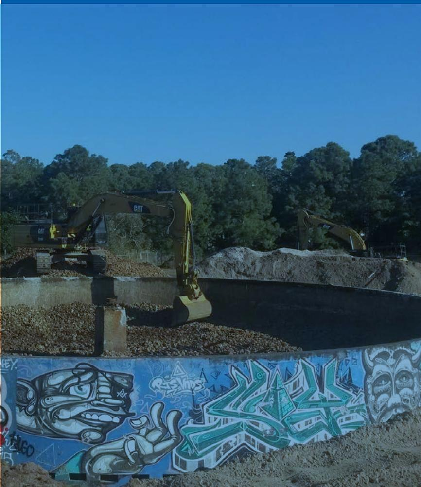
Liberty has excavated identified “hot spots” from the Remediation Action Plan and disposed to landfill up to 2,000 tonnes on asbestos impacted soils, including waste from the former “grit and rag” location.
